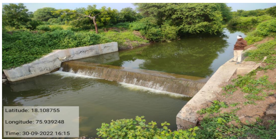
Figure 28: Cement Nala Bund constructed in Walgud Village, Dharashiv
