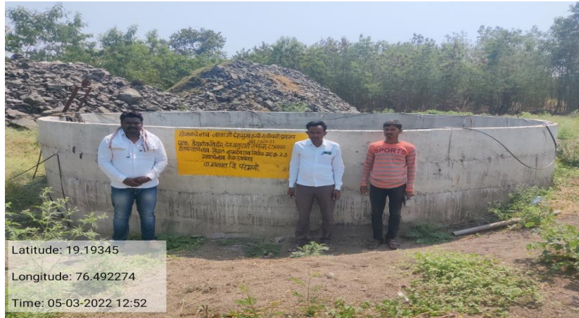
Figure 30: Open Dug Well in Project Area in Parbhani
